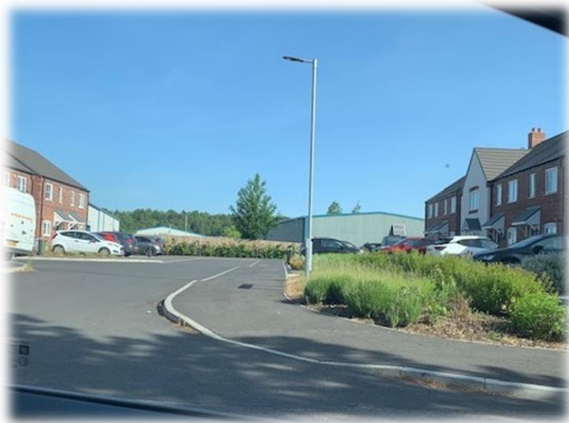
Figure 4: View towards centre of development highlighting over dominance of front of plot parking
