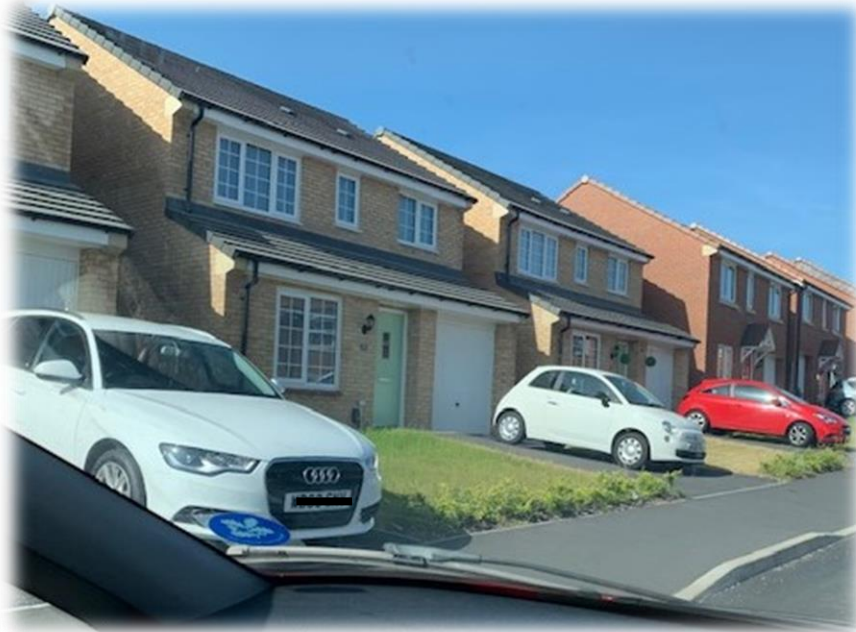
Figure 21: View of integral garages in the development
