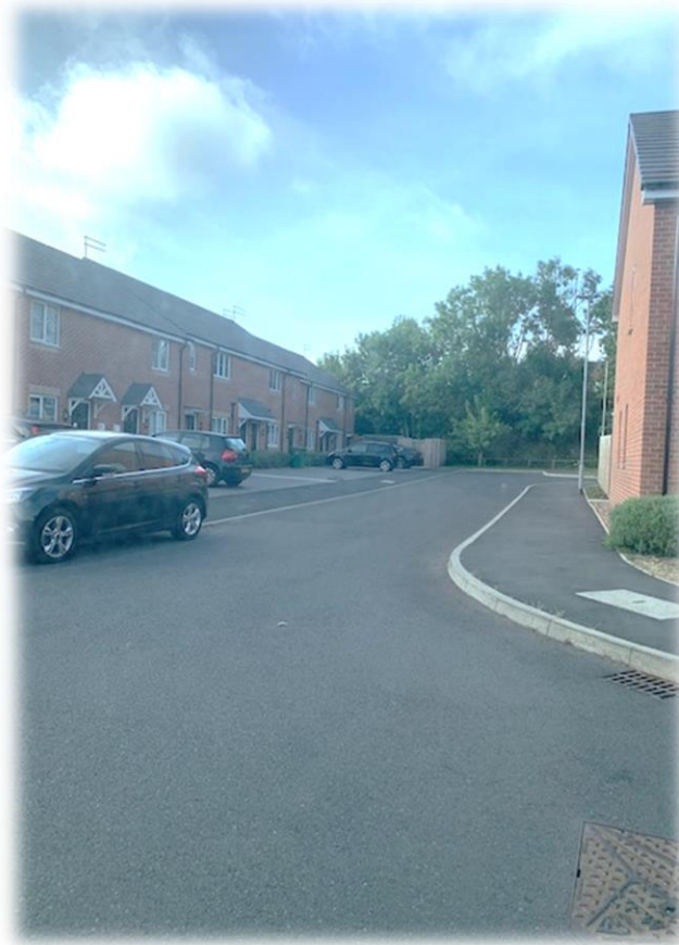
Figure 15: View of the development
